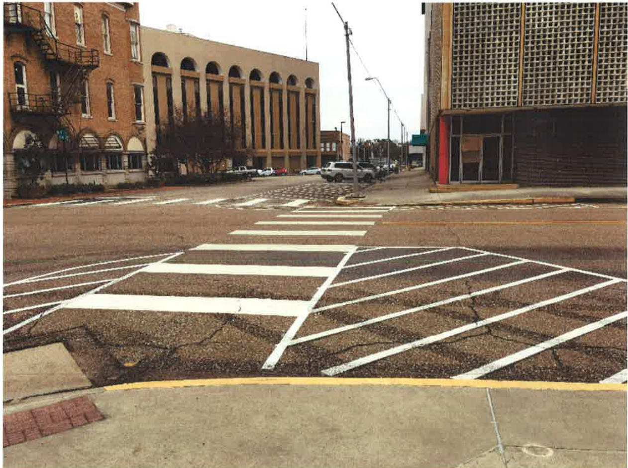
More visible crosswalks with painted bulbouts to slow vehicular turning speeds now connect existing sidewalk infrastructure downtown and improve safety and walkability.
